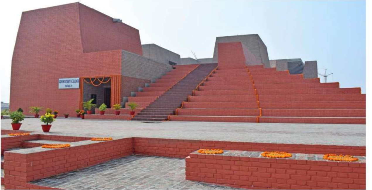
Administrative Block | Wing - 1
