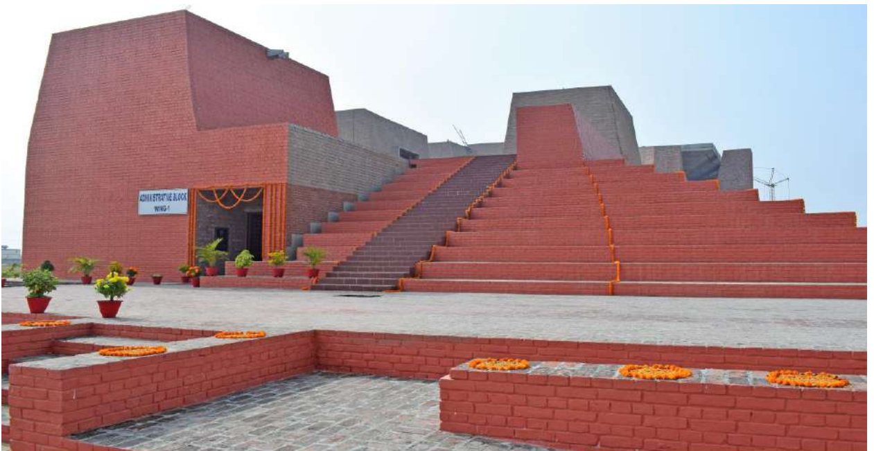
Administrative Block | Wing - 1
