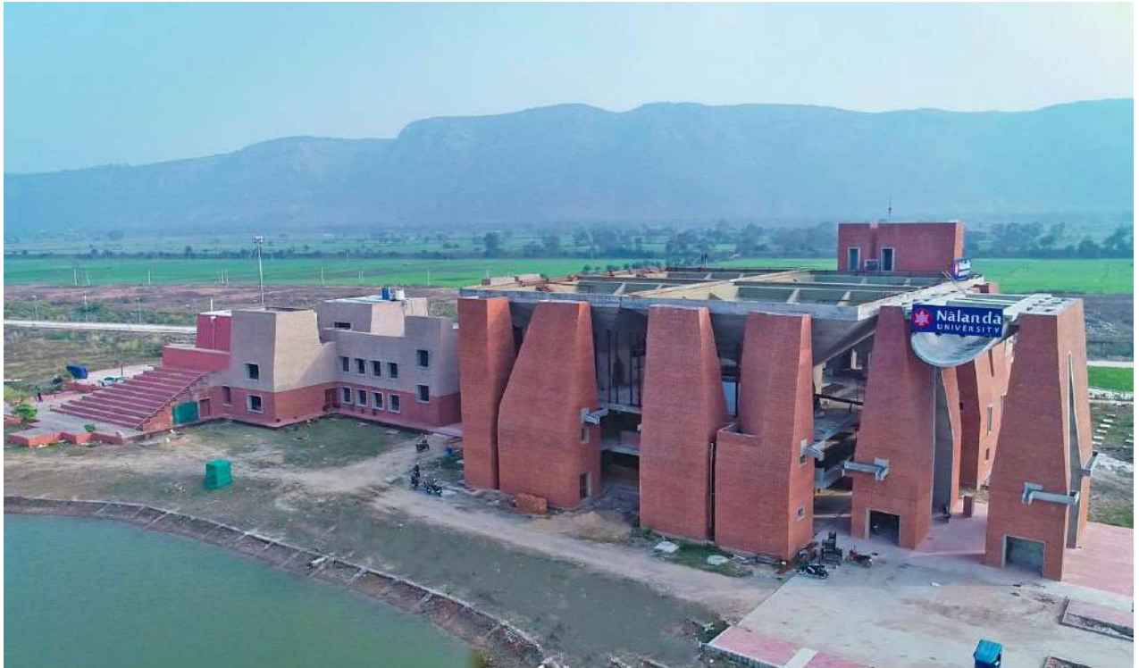
Aerial View of Admin Block
