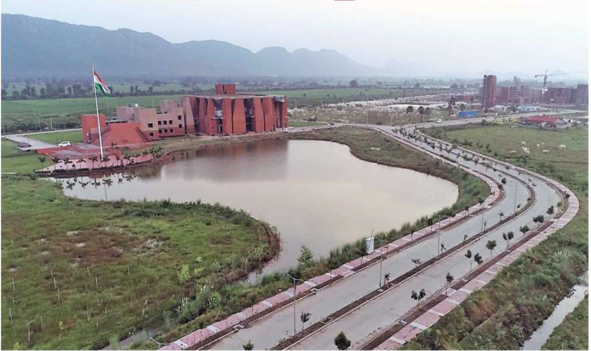
Aerial View of Administrative Block with Water Body
