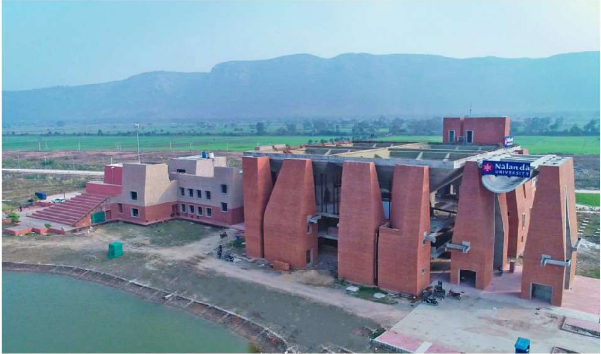
Aerial View of Admin Block
