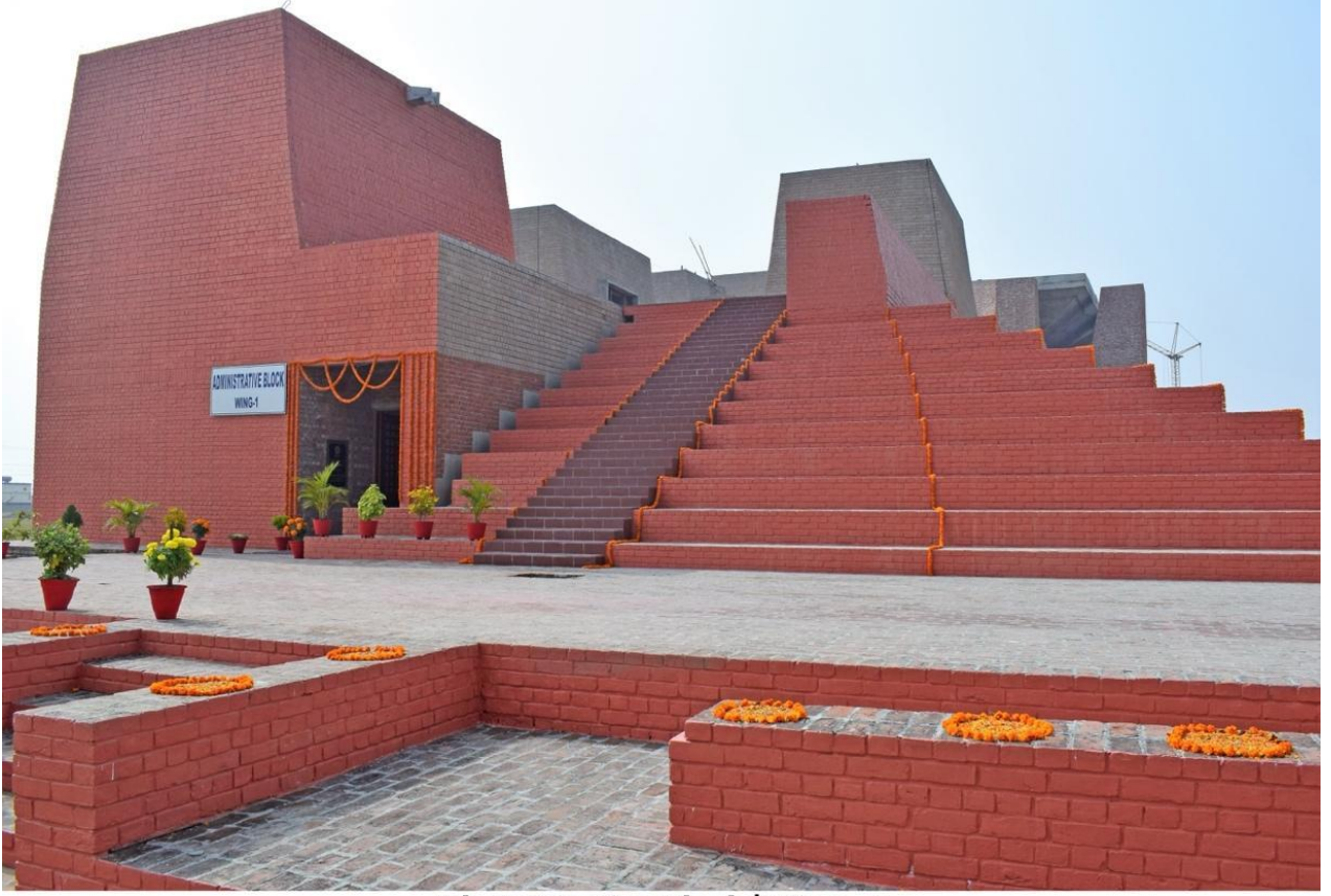
Administrative Block | Wing - 1
